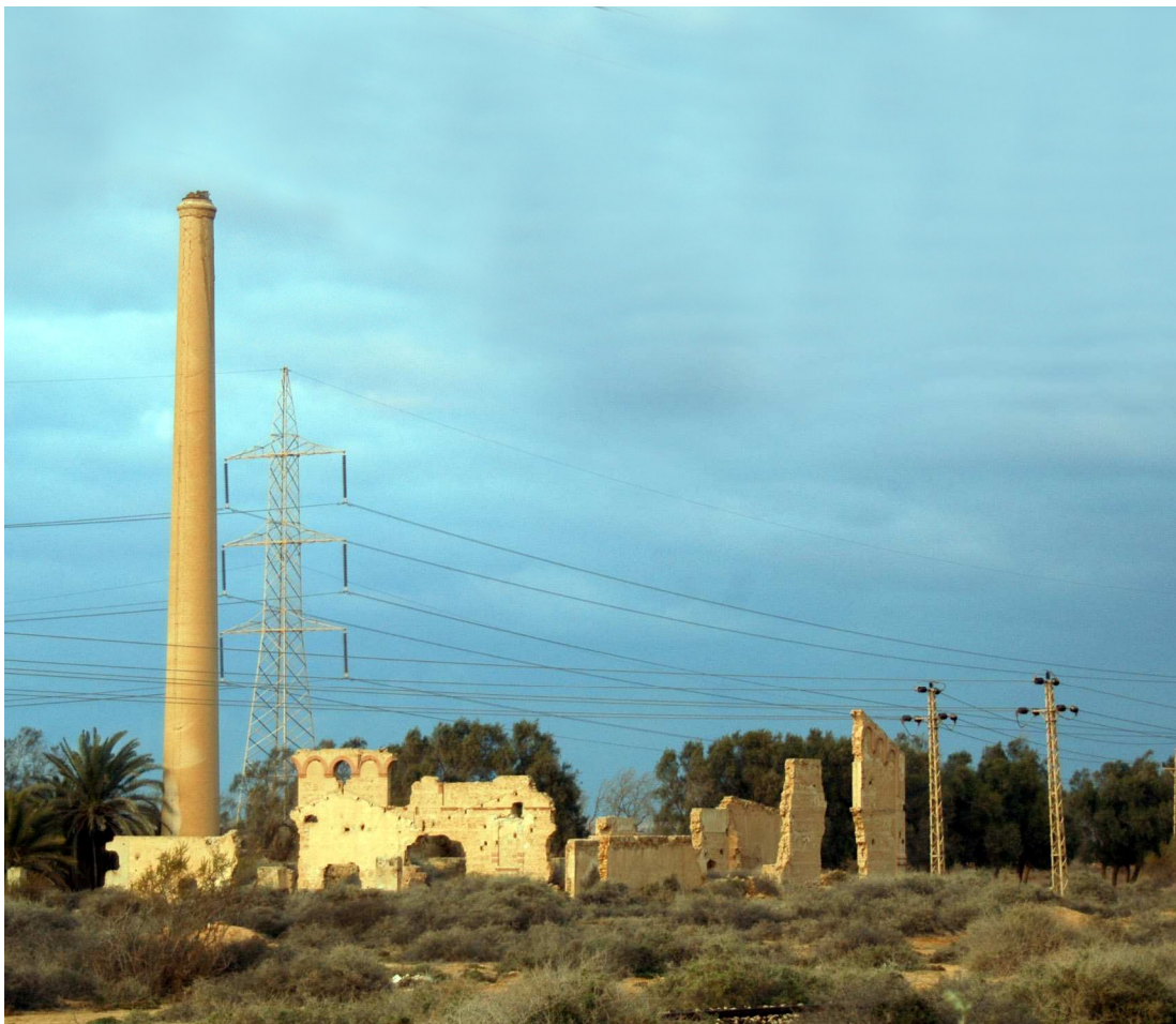
Neglected Clay Factory in El Hammam village West of Alexandria
